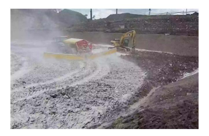
2. Cement: Cement is another commonly used chemical stabilizer. When added to the soil, it reacts with water to form cementitious compounds, which bind the soil particles together, increasing its strength and stability.
